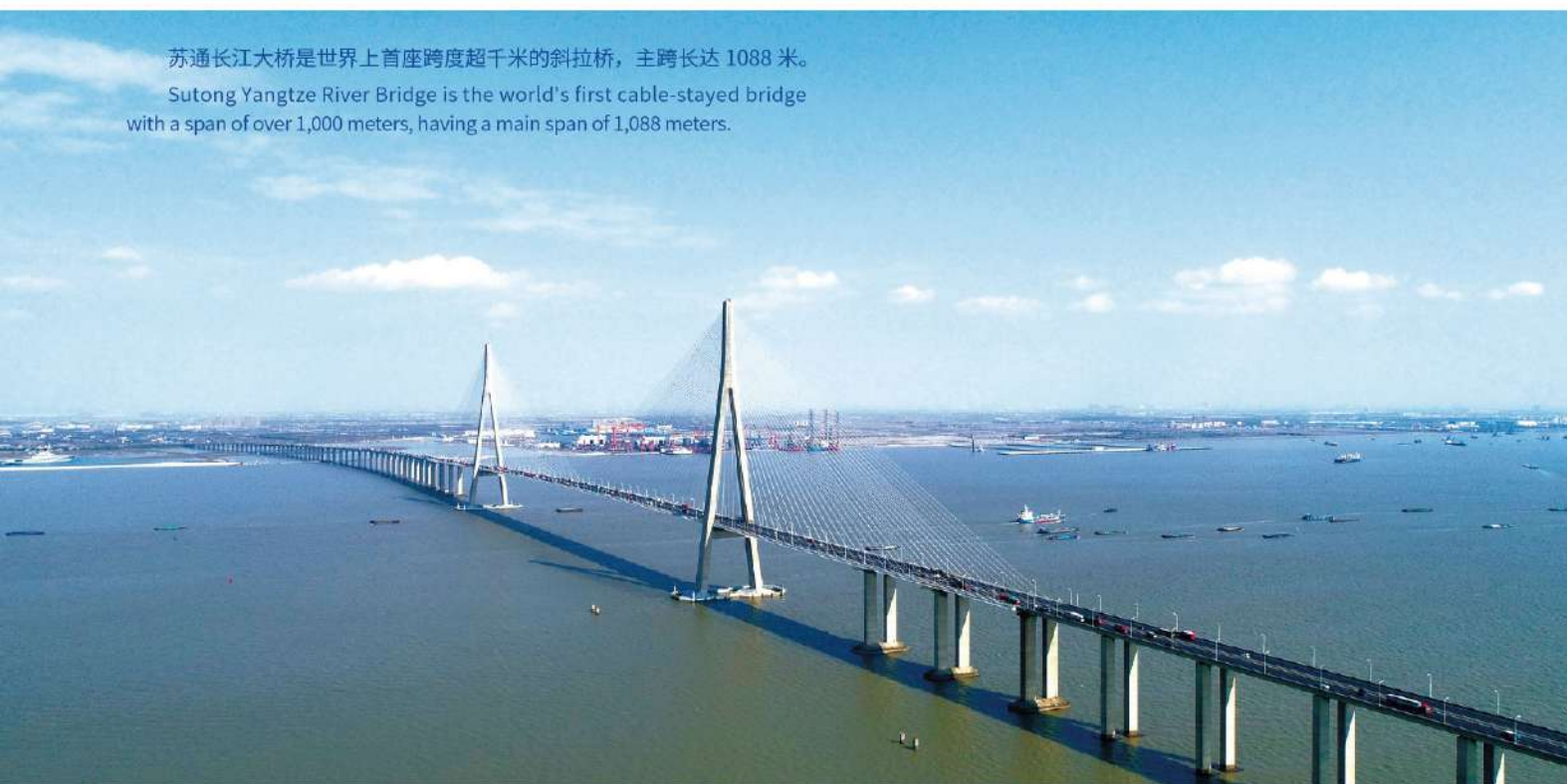
苏通长江大桥 Sutong Yangtze River Bridge
