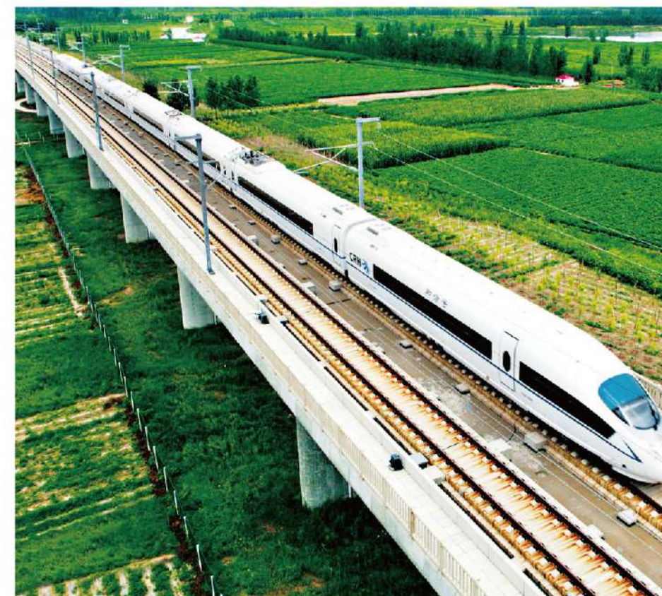
京沪高速铁路 Beijing-Shanghai High-speed Railway
