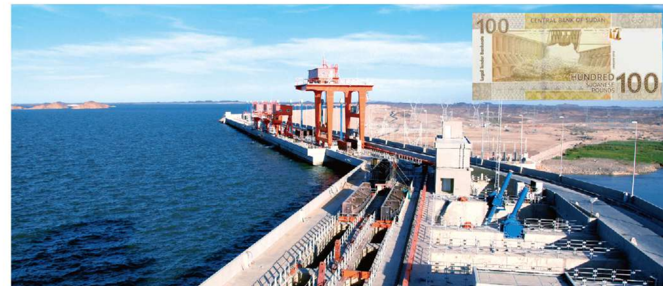
苏丹麦洛维大坝 Merowe Dam, Sudan
