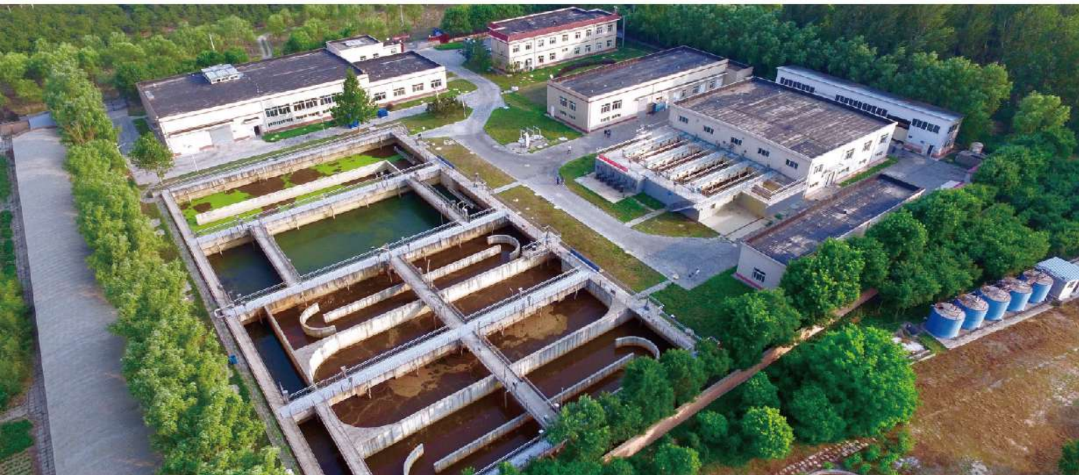
北京翠湖新水源厂 Cuihu New Water Source Plant in Beijing
