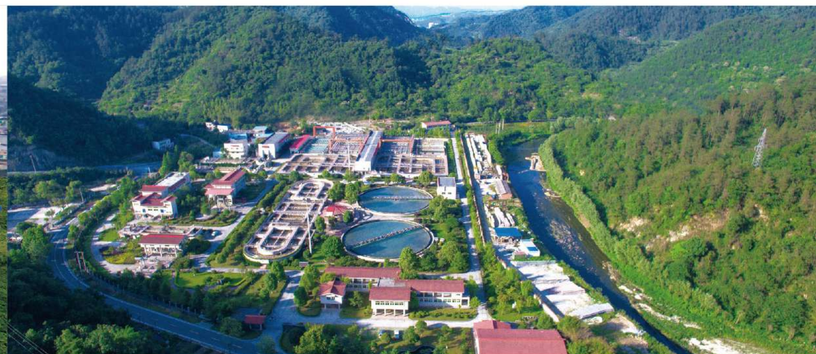
湖北十堰神定河污水处理厂 Shen-Ding River Swage Treatment Plant at Shi-Yan City, Hubei Province
