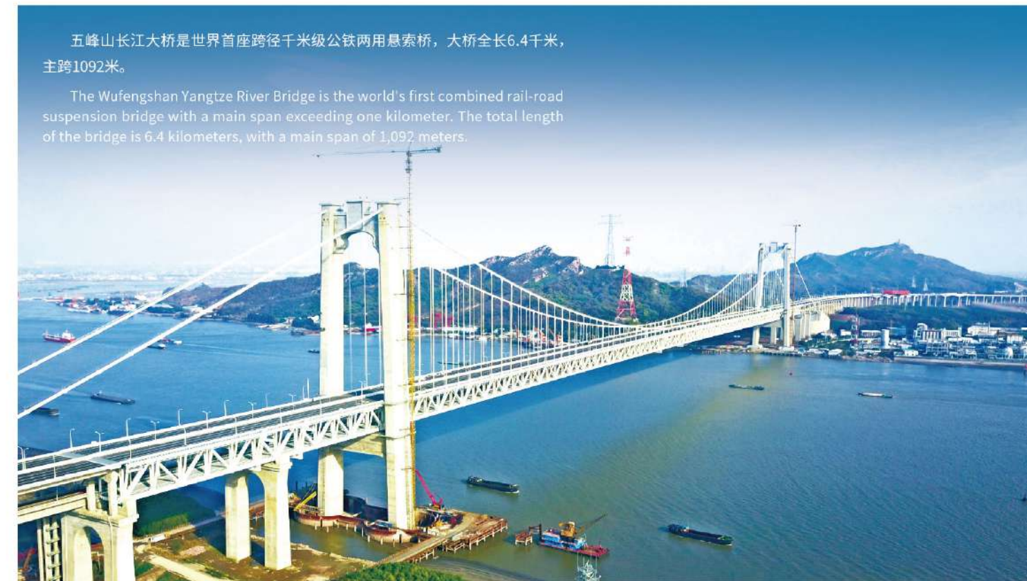
五峰山长江大桥 Wufengshan Yangtze River Bridge
